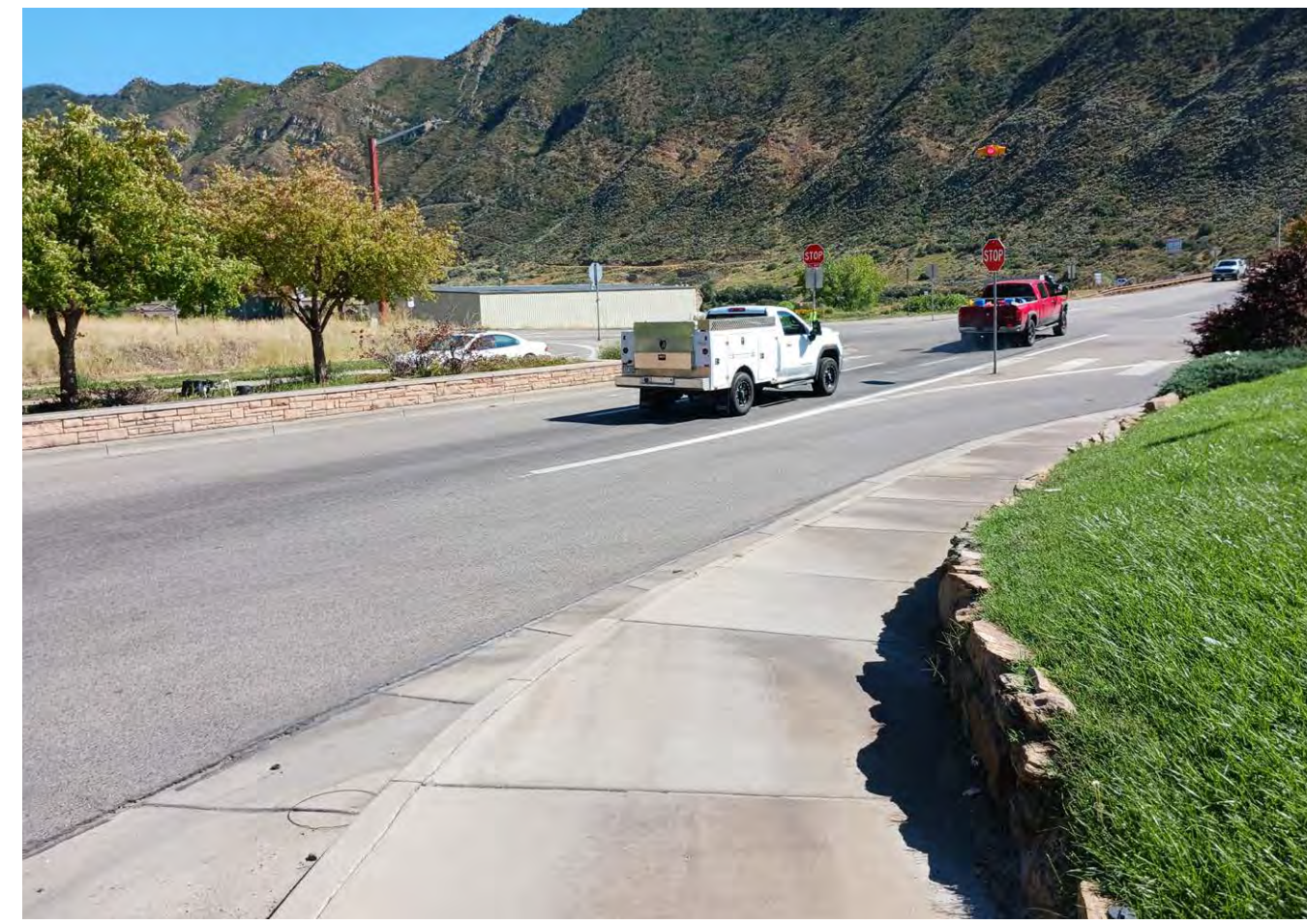
2. View of the intersection facing South.
